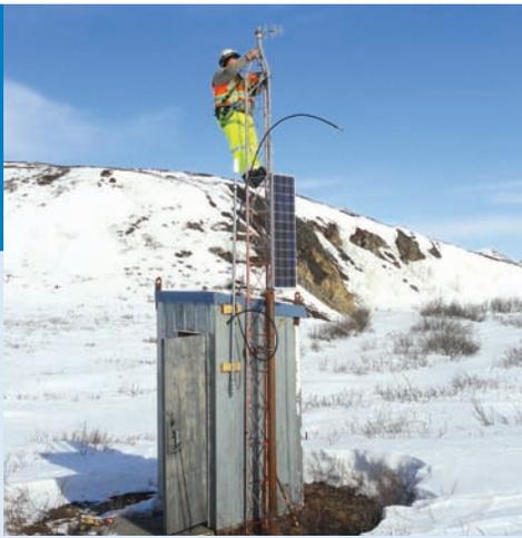
*Dennis Sheldon changing the cable for the radio antenna. The radio is used to send data from the stream station to the Pi System.*
